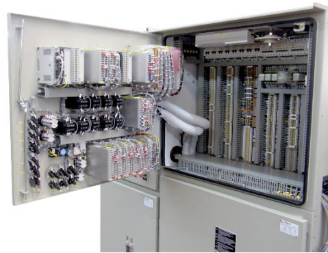
Figure 83. Inside of the LV compartment
