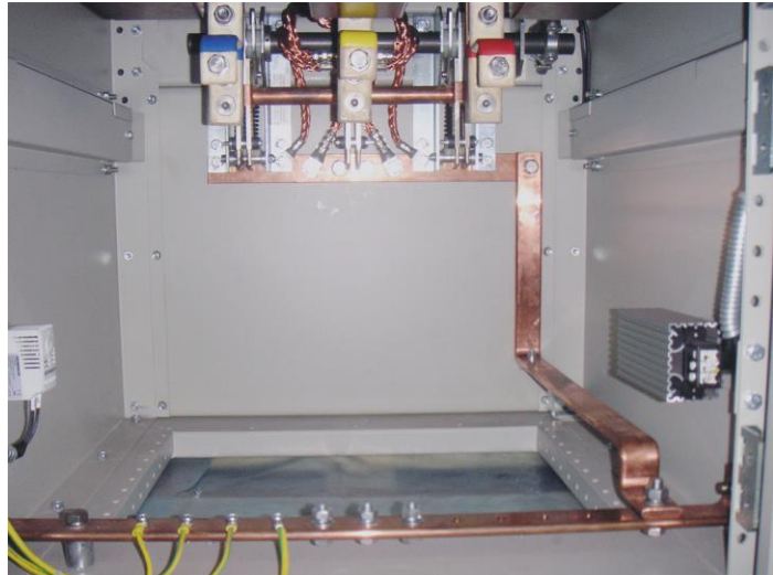
Figure 61. Cable connection compartment
