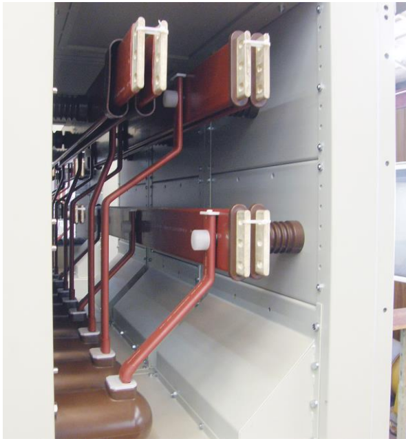
Figure 9. Busbar compartment
